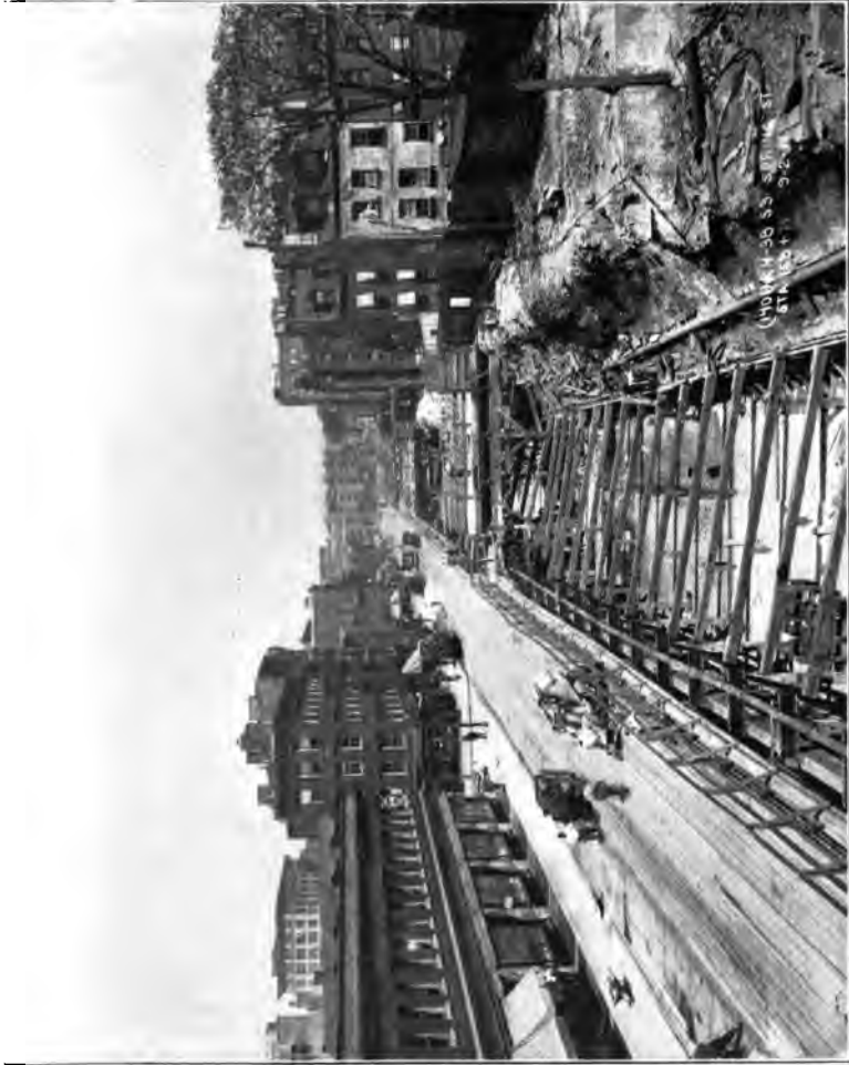
Photograph kindly furnished by Public Service Commission, First District, New York Illustration No. 8. —Yarlick street, New York City, was recently widened from 65 feet to 100 feet by taking 35 feet from one side of the street, as shown in the illustration. A new subway line is now being constructed. This is an example of street improvement which St. Louis must soon undertake. The irregular building line caused by the widening of the street demonstrates the need of excess condemnation for such improvements.
